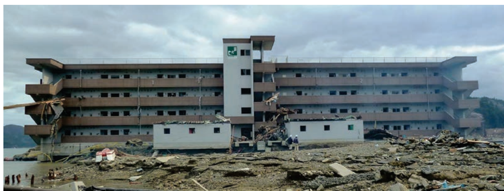
Figure 6-2 Reinforced concrete apartment building designated as a vertical evacuation structure in Minamisanriku, Japan, 2011 Tohoku tsunami.
