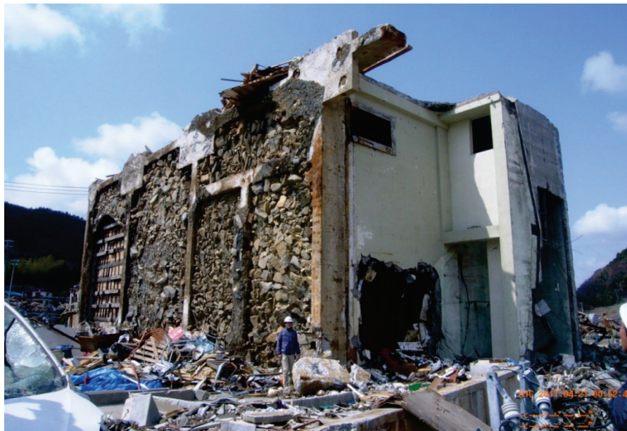
Figure 2-28 Overturned cold storage building in Onagawa, Japan, 2011 Tohoku tsunami (photo courtesy of G. Chock and ASCE, from Chock, et al., 2013b).
