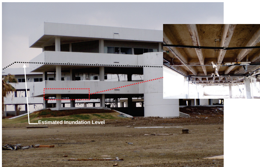
Figure 2-31 Office building in Pass Christian, Mississippi, with a cast-in-place concrete pan joist floor system that suffered nonstructural damage in the first two stories, but no structural damage, 2005 Hurricane Katrina (photos courtesy of I. Robertson).
